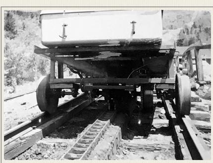
View of down hill end showing suspension, cog gear, brake drum, etc. (1976) - Walter King photo / NH DOT archives
