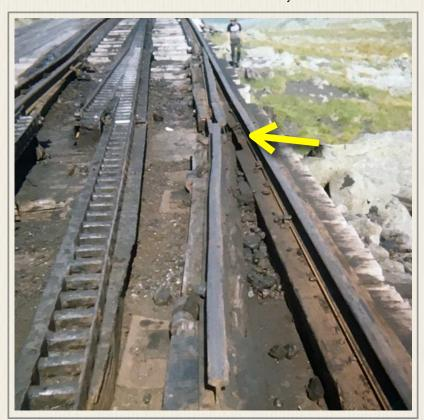
**Photo No. 4:** Down-mountain view of Skyline Switch for movement from siding. Note misalignment at upper center (1979)
