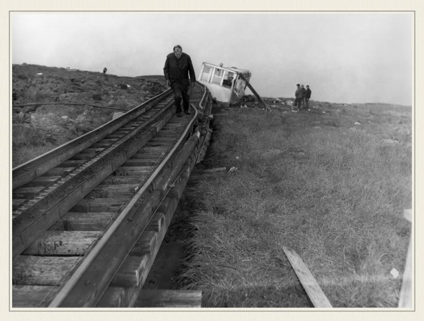
"The main force of the collision appeared to be caused by striking a jagged rock at the right front corner of the car. The right side of the car was damaged and windows broken. The front end remained intact with two windows to the right of the center broken and the two to the left of the center remaining un-cracked.
