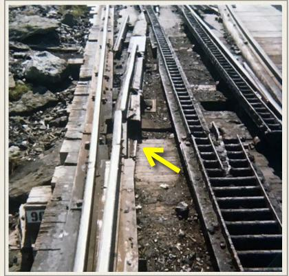
**Photo No. 2:** Up-mountain view of Skyline Switch partially set for siding. Note misalignment at left center (1979)
