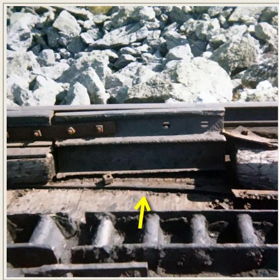
**Photo No. 6:** Closure rail at Skyline Switch. Note broken weld at base of support. (1979)
