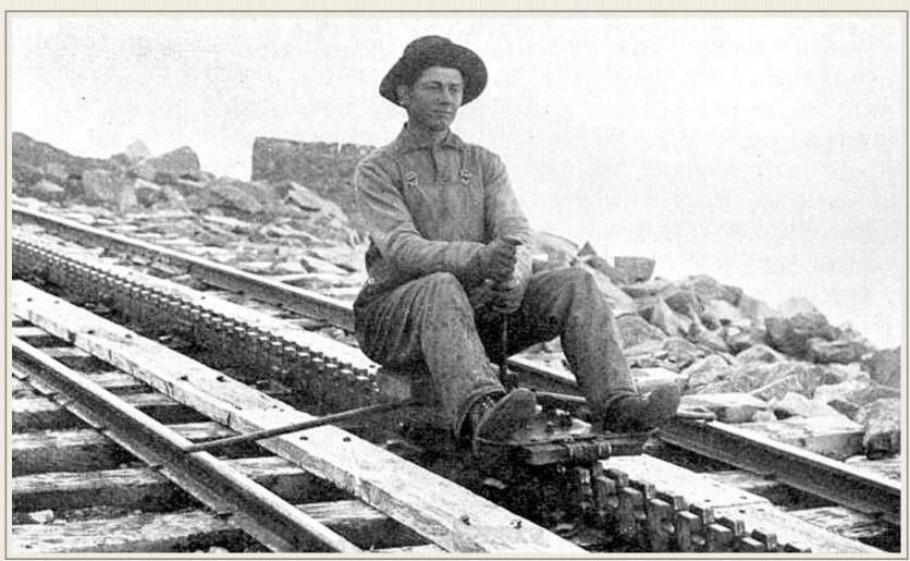
Pike's Peak - Similar, But Different: The Colorado cog railway was of a similar, but different design - both in the center cog rack, and the workers' "hand cars" to descend the line. The western boards were not as wide and ran outrigggers to the outside rails for stability. (1904)
