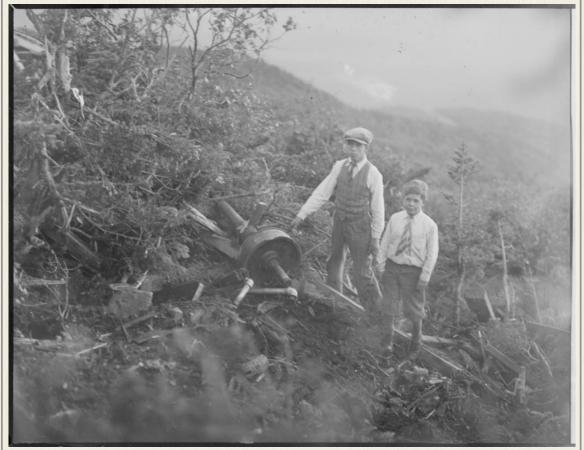
of the engine sufficiently to disengage the forward cog from the rail, and when this end of the engine came down the cog wheel failed to mesh with the cog rail."
