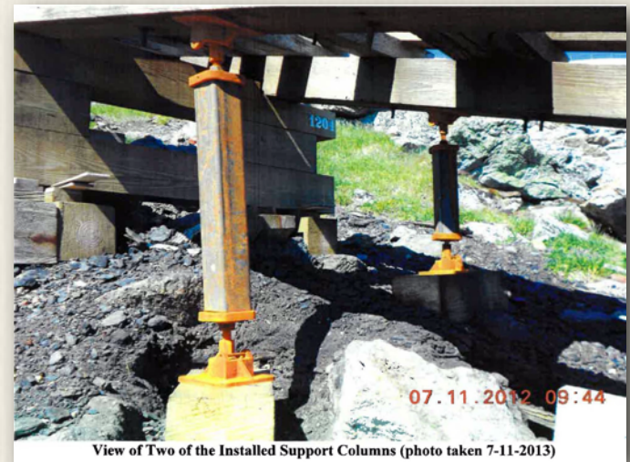
View of Two of the Installed Support Columns (photo taken 7-11-2013)
