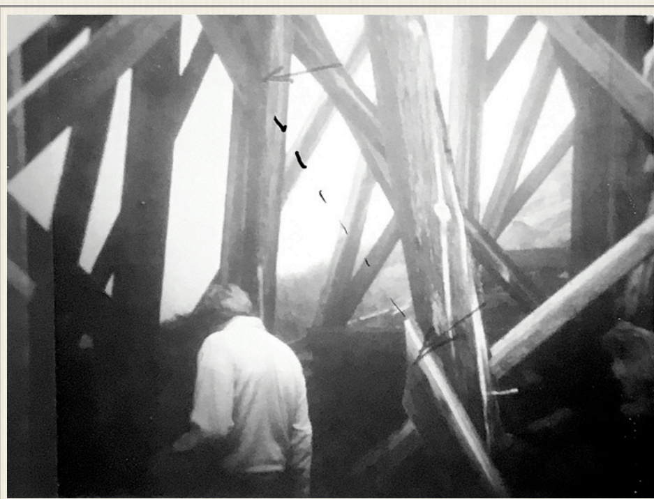
NH Bridge Design Bureau personnel inspect Bent 680 - finding diagonal bracing cut out, right side as indicated by dotted line on photo (May 1986) - NH Transportation Dept files
