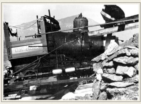
moved and the engine was rolled over onto its wheels (above) onto a temporary trestle. The engine was then pulled up onto the trestle via the temporary trestle, and was taken down the track to the repair shop at the Base. It is interesting to note that only one of the four cylinders of the engine was damaged, the engine was taken down the tracks under its own air compression (below) and it was not necessary to use any other engine or equipment to brake the speed of the damaged locomotive."
