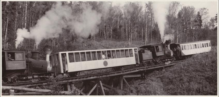
This exclusive Courier photo shows the Mt. Washington Cog Railroad's new aluminum and steel passenger car as it made a brief appearance outside the car shops this week. Still under construction, the car will be placed in use next season, the first of several the line expects to construct which will eventually replace the wooden cars now in use on the famous mountain ride. Its trim lines can be compared with that the conventional wooden car on the train ahead (Oct 1957) - Photo by Presby
