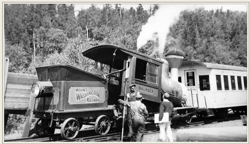
Cog crew kibitz at the fill pipe as No. 9's tender is filled with water at Base Station. Note the tender light for moonlight service
