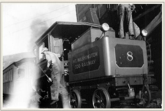
Engineer Cliff Kenney swings down from the cab of the Tip Top to lubricate his engine.
