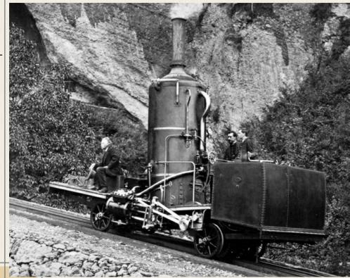
**Above:** Engineers Niklaus Riggenbach (seated front) and Olivier Zschokke test driving a cogwheel steam locomotive for the Vitznau-Rigi Railway on Mount Rigi in Switzerland (circa 1870)
