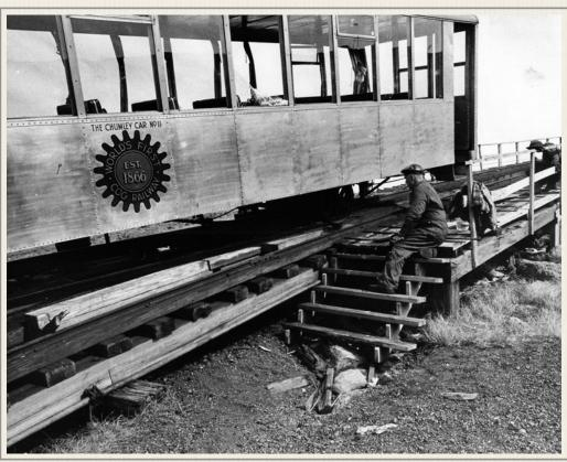
Back on the tracks the ill-fated Chumley Car No. 11 is given a final undercarriage check before descending the mountain. The under-carriage and braking system were in perfect condition and made the descent without incident. (1967)
