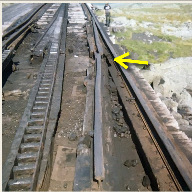
Photo No. 4: Down-mountain view of Skyline Switch for movement from siding. Note misalignment at upper center (1979) - King photo / NH Transportation Dept.
