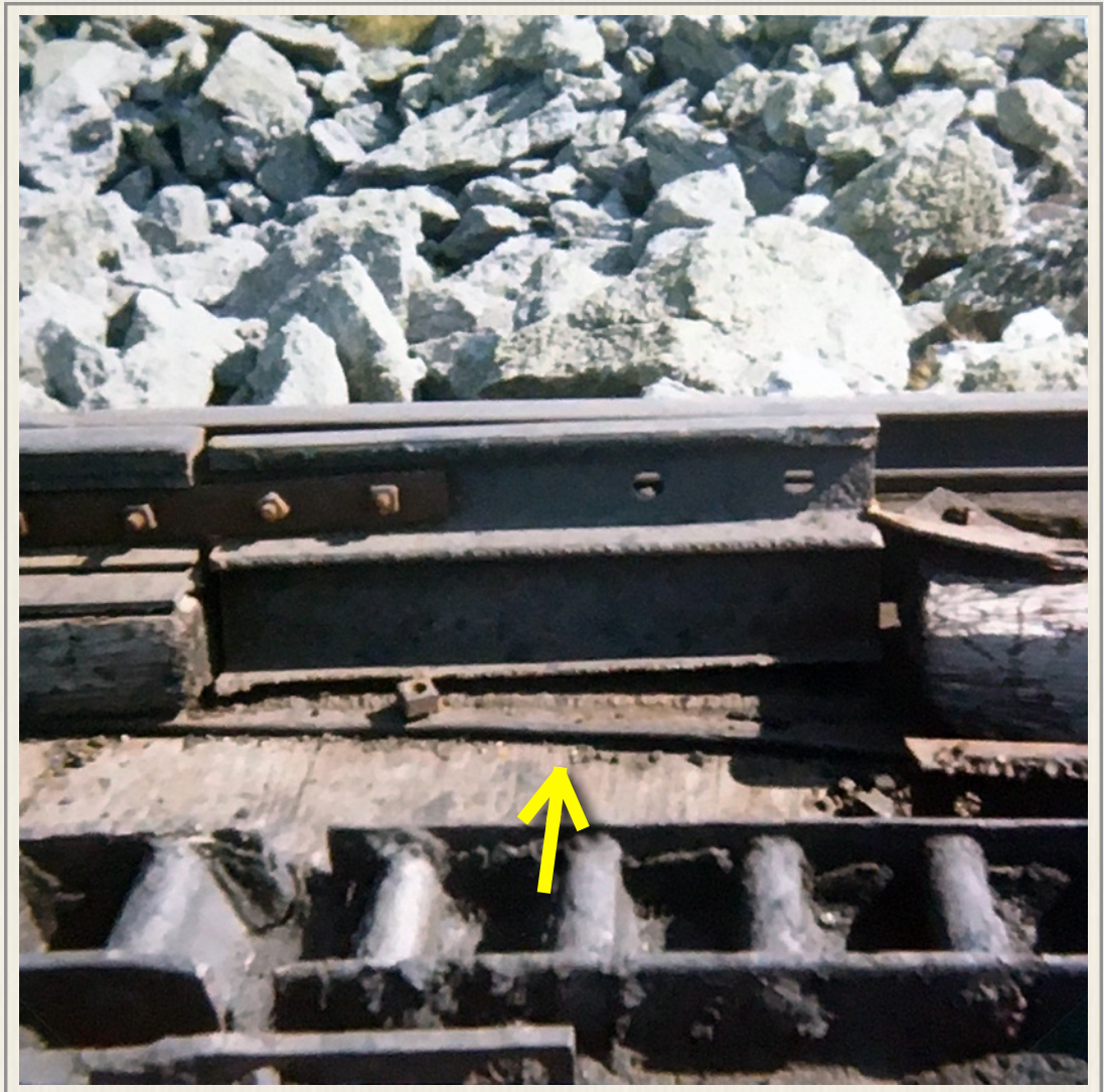
Photo No. 6: Closure rail at Skyline Switch. Note broken weld at base of support. (1979) - King photo / NH Transportation Dept.
