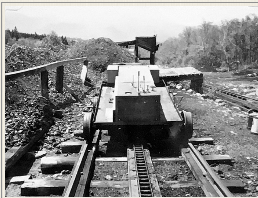
View of the up hill end of "Speeder" - Controls are on the uphill end (1976) - Walter King photo / NH DOT archives
