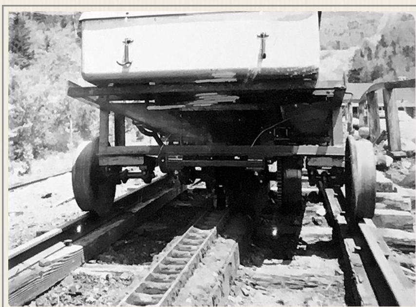
View of down hill end showing suspension, cog gear, brake drum, etc. (1976) - Walter King photo / NH DOT archives
