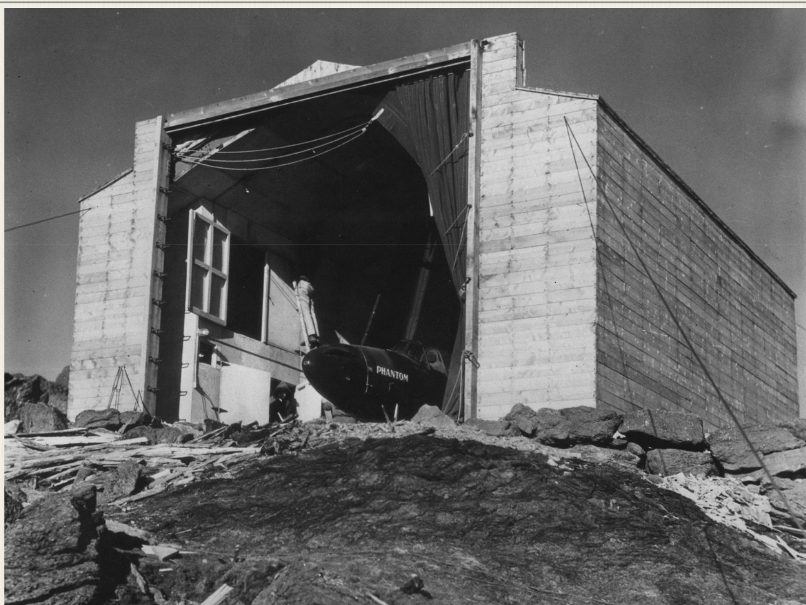
The Phantom's Winter Lair: Icing test hanger atop Mount Washington, New Hampshire, looking northwest, before the winter season closed down. In portion of shed to left, the auxiliary power unit, which is a motor-driven electrical generator, is in the upper level and the ground heater room is on the lower level. This picture shows the steel cables which secured the hanger to the rocky mountainside. Biggest problem was the canvas curtains strung across both ends of the "wind tunnel." (1947) - US Navy photo / Lewis Family Collection
