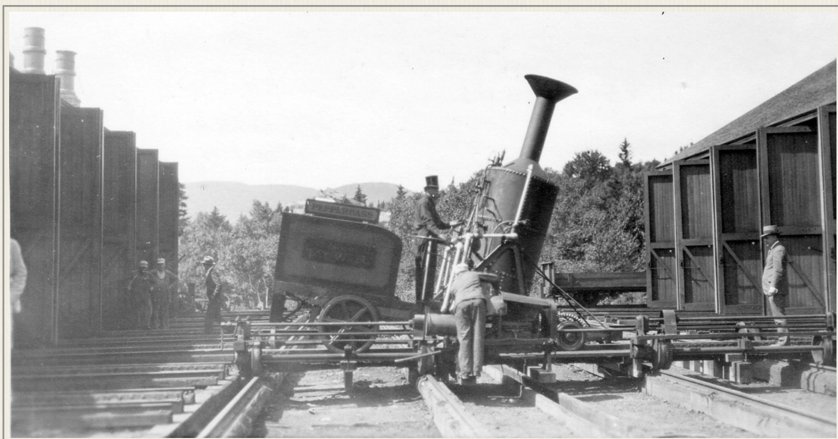
Old Peppersass is run out onto the transfer and moved to the mainline to run up to its re-dedication celebration. The photo shows the Model-T engine rigged to move the transfer back and forth. (July 20, 1929) - B&MRR Historical Society Collection
