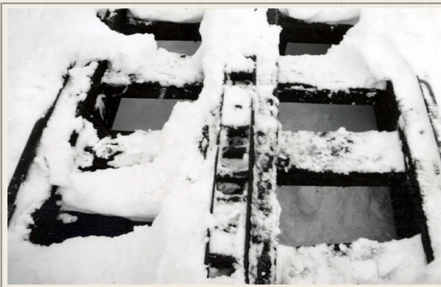
Snow covered cog track showing reduction gear clearance (Mar 1952) - Davenport-Besler photo
