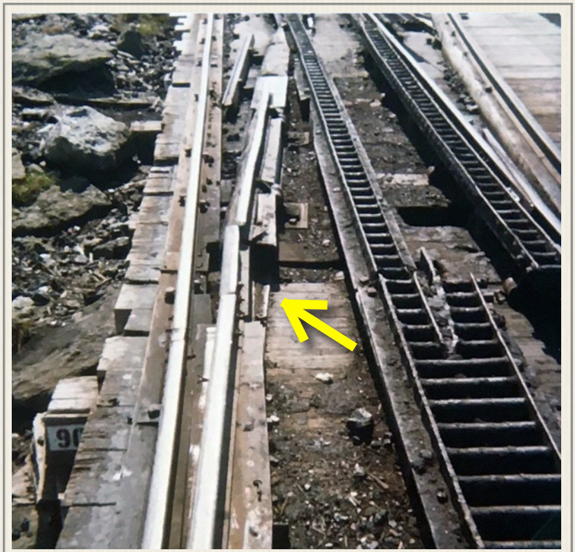
Photo No. 2: Up-mountain view of Skyline Switch partially set for siding. Note misalignment at left center (1979) - King photo / NH Transportation Dept.
